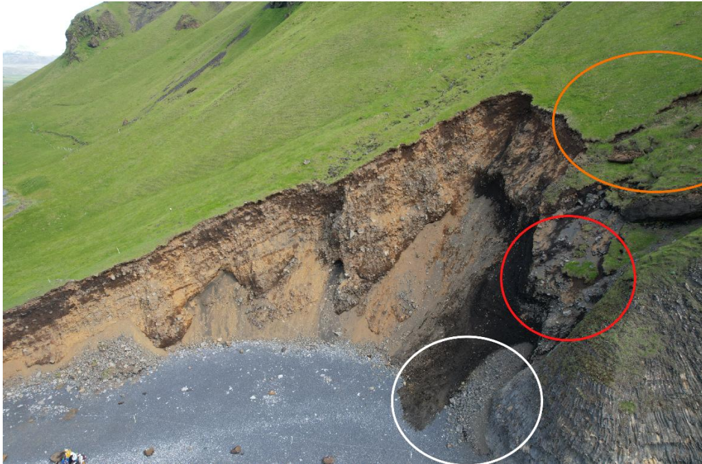
Figure 9 the erosional scarp in Reynisfjall mountain. The red ring shows the active part of the scarp and the white circle is where the material ends up. An old scarp that until now has remained stable and is marked with an orange circle.
