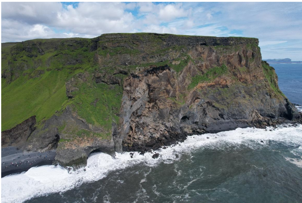
Figure 13 shows the new rock collapse from Reynisfjall mountain. The photo was taken on the 3 rd of July 2026.
