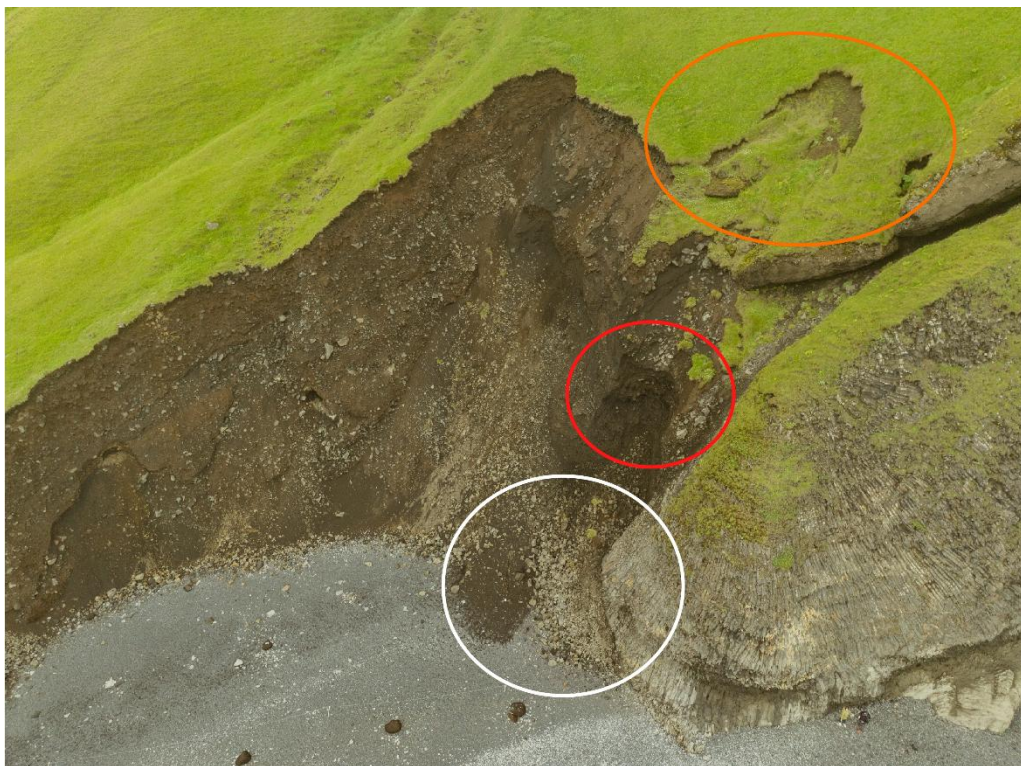
Figure 10 the erosional scarp in Reynisfjall mountain. The red ring shows the active part of the scarp and the white circle is where the material ends up. An old scarp that until now has remained stable and is marked with an orange circle.
