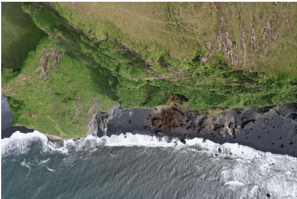
Figure 10 shows the cliff face of Reynisfjall and the beach below. The photograph was taken at 10:55 on 15 th of June. There is fresh debris on the beach and a new scar in the cliff can be seen as well.
