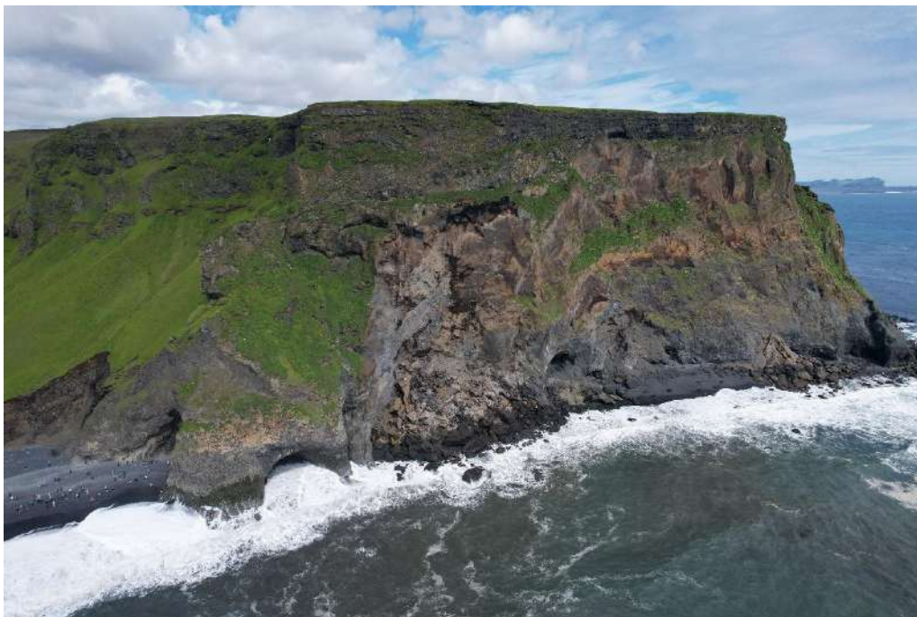
Figure 12 shows the new rock collapse from Reynisfjall mountain. The photo was taken on the 3 rd of July 2026.
