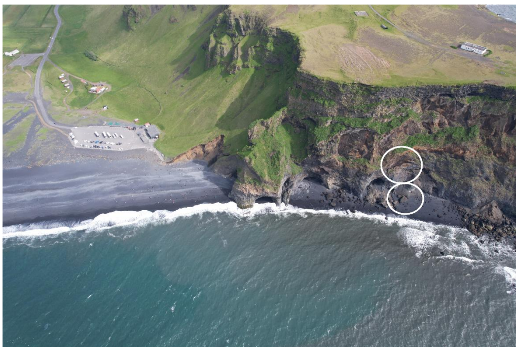
Figure 13 is a photo taken on the 15th of June, where the ledge (upper white circle) has broken off from the cliff and there are three large rocks on the beach below (lower white circle).
