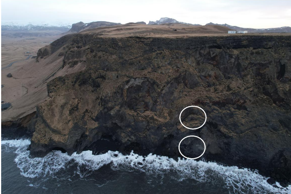
Figure 14 is a drone photo that was taken on the 11th of February, where the ledge (upper white circle) is still attached to the cliff and there are no large rocks on the beach below (lower white circle).
