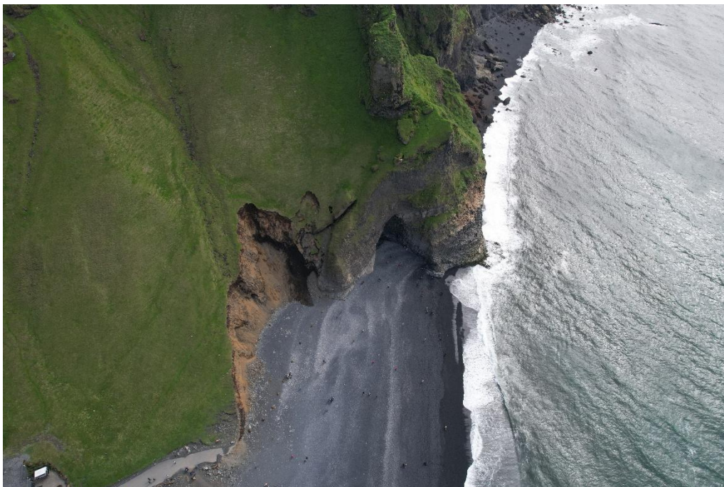
Figure 7 shows the erosional scarp into Reynisfjall, the basalt columns and the cave, along with the beach itself. Before the erosion event in 2026, the beach extended well beyond the basalt columns and the eastern part of the beach was easily accessible.
